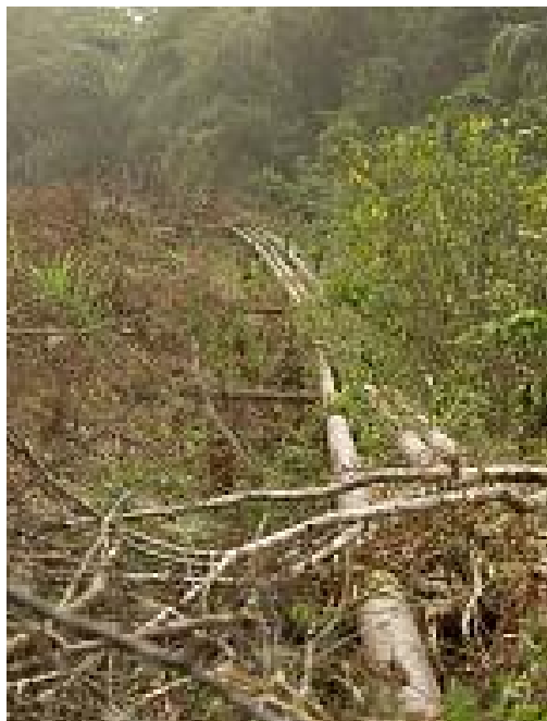
Pipelines now part of sustainable development at the World Bank
